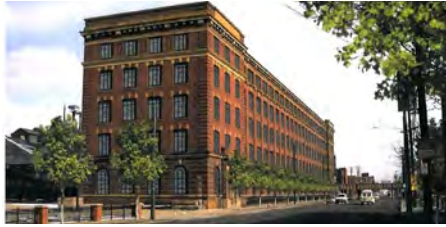
WARNER & SWASEY REDEVELOPMENT Underway
